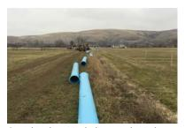
Completed a 12-inch diameter buried pipeline that is 1,960 feet long and serves six landowners in the Manastash area.
